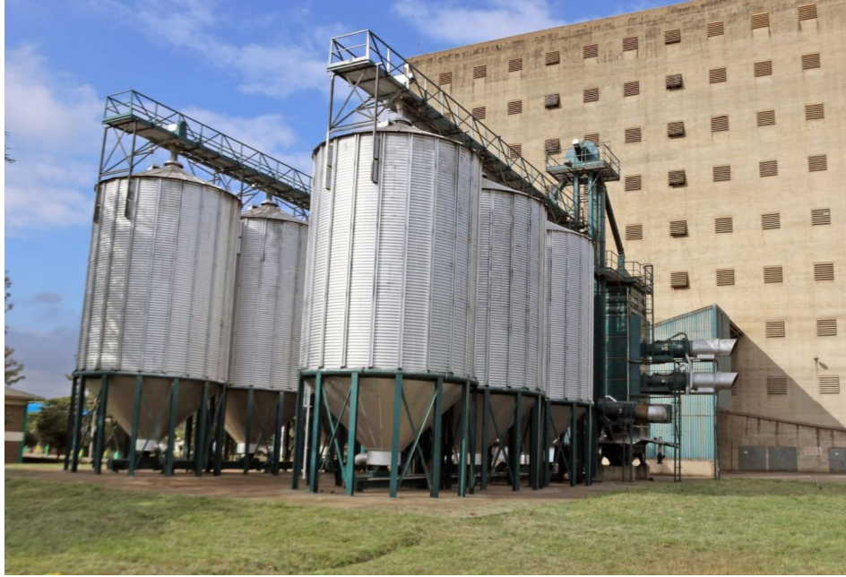
Plate 4-4: Infrastructure for Drying of maize at a NCPB warehouse Source: Author (2023)
