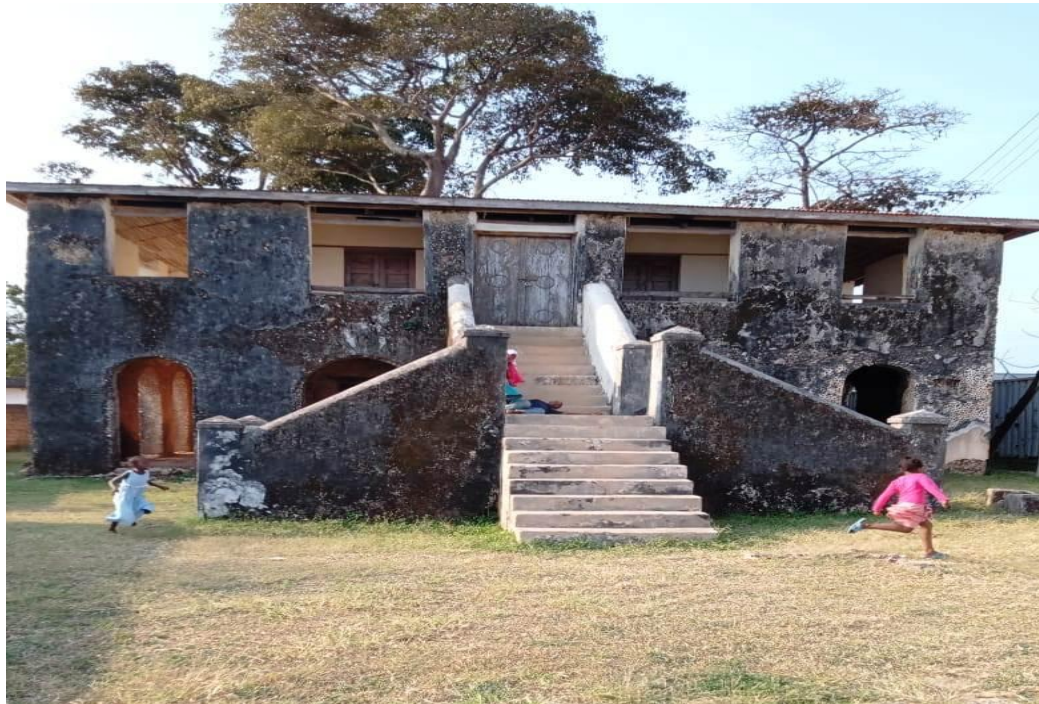
Plate 11: IBEACo administration building exposed to human interference
