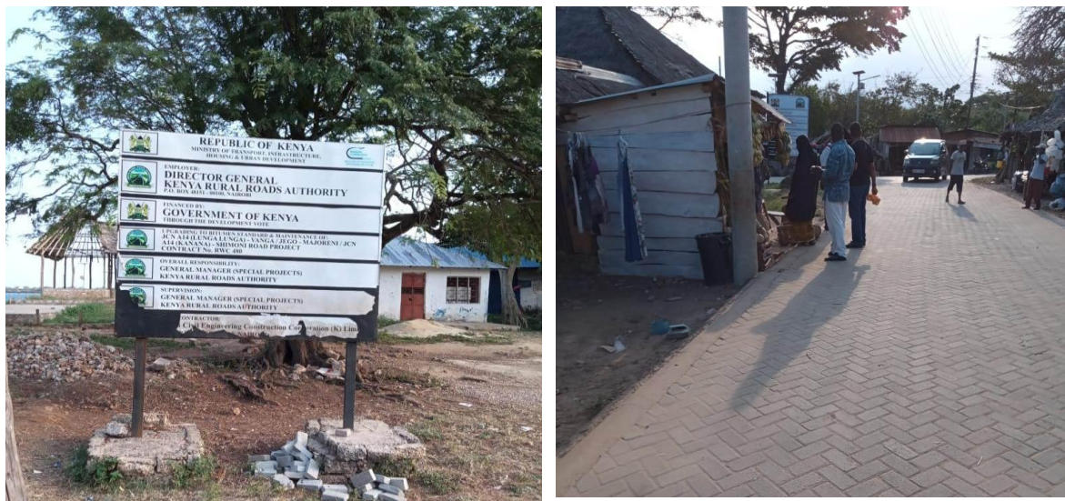
Plate 17: Road construction through Shimoni town, a project by KERRA
