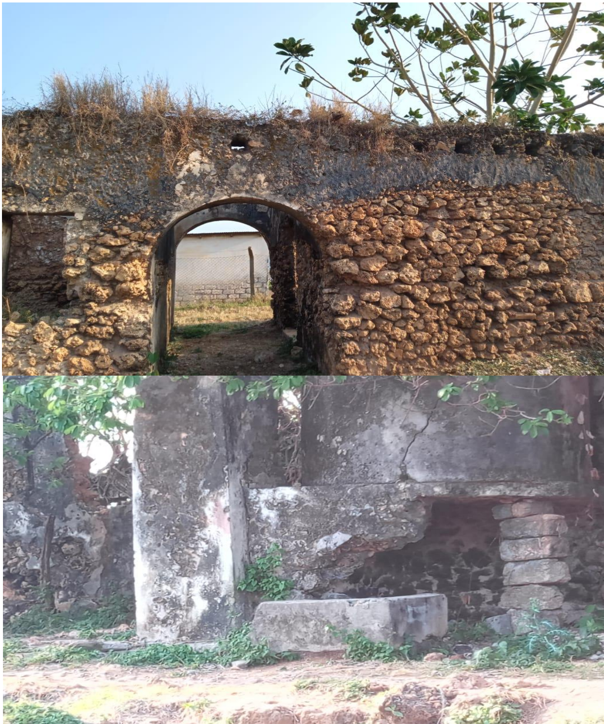
Plate 14: Threat of Vegetation forming a canopy and drilling in to the walls at Shimoni caves and colonial prison respectively
