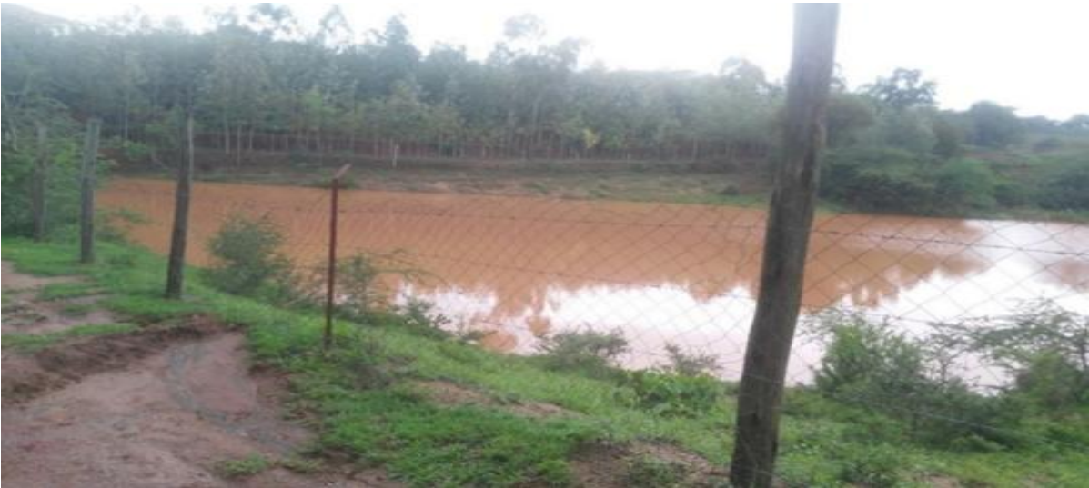
Plate 2: An Earth Dam at Kwa Mutuku Village constructed through the support of the project to address water shortage
